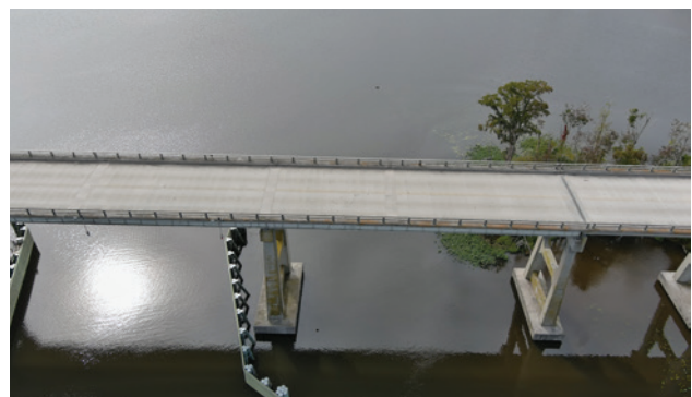
Existing Conditions at the BRITE Bridges
